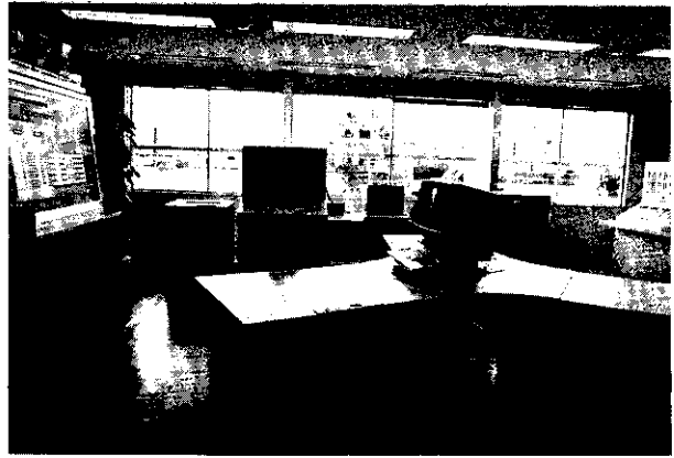
Photo 1 View of Control room
